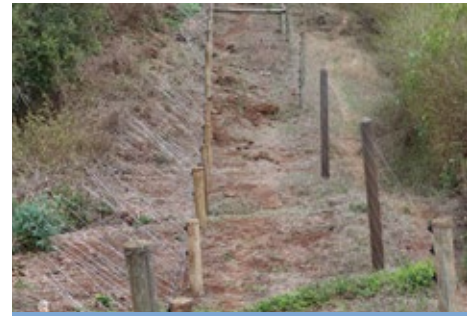
Short fence constructed in front of the main fence to deter elephants' interference
