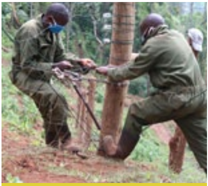
Team work - straining tightlock mesh
