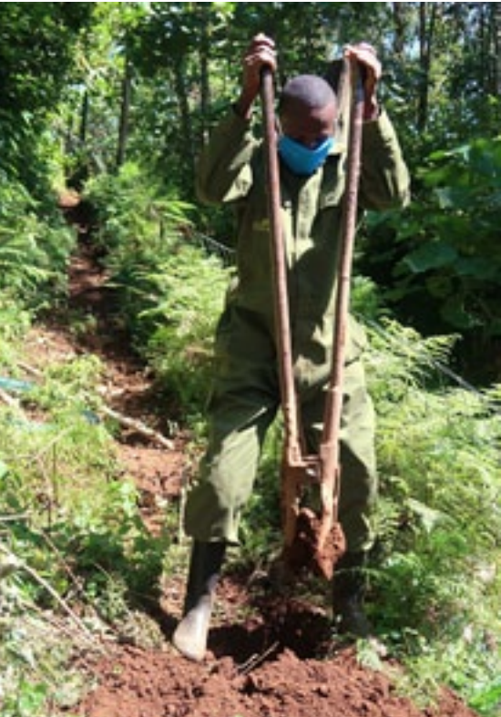
Fence attendant digging a hole for a fencing post using a hole digger
