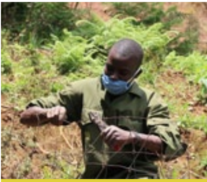
Joining tightlock mesh wire
