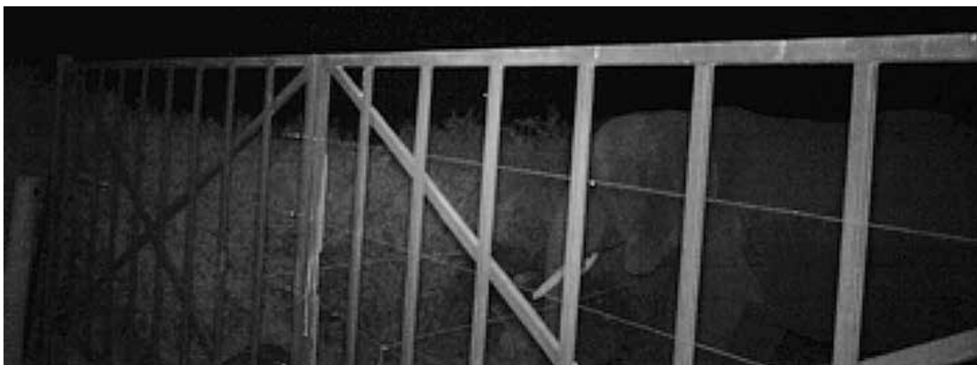
The one-way elephant gate won't open when the elephant approaches it from inside the forest. This means no elephant exits the forest through the gate.
