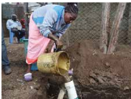
Adding dung mix to digester
