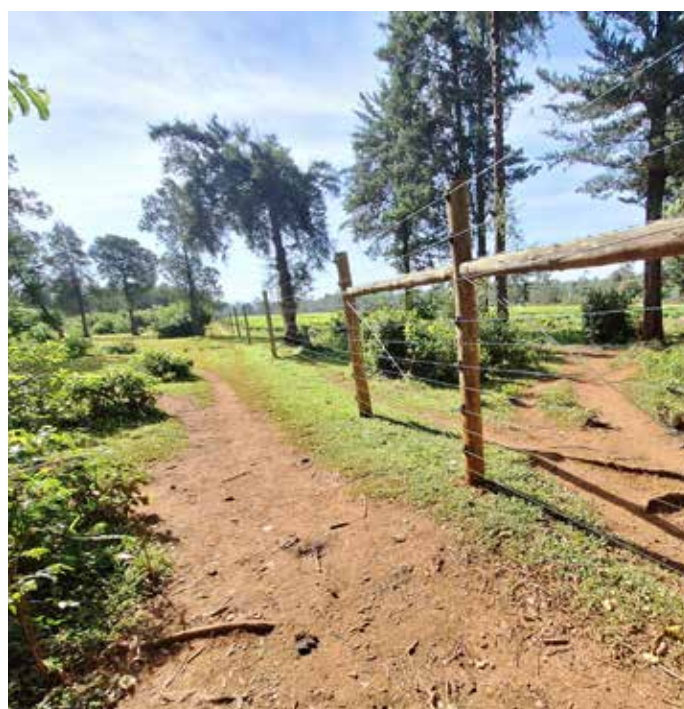
Completed section of the Kakamega electric fence
