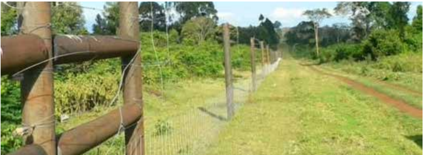
A section of the Mount Kenya comprehensive electric fence line.
