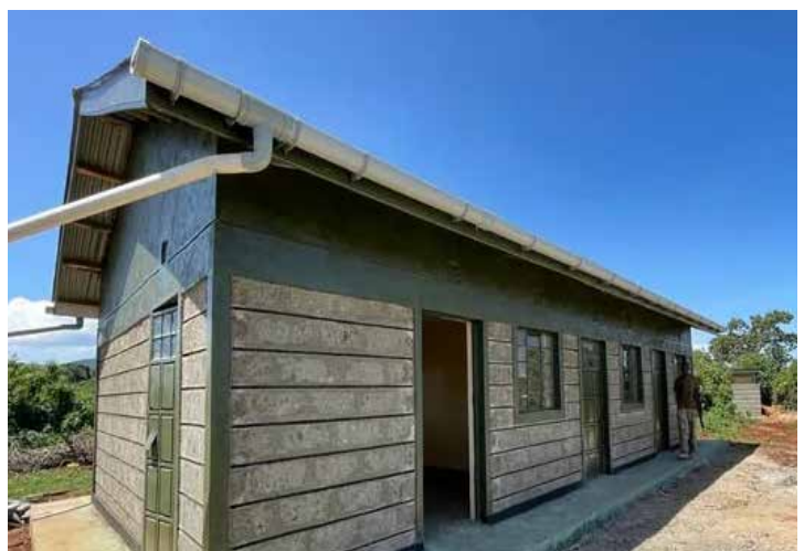
Black Rhino fence energizer house in the Aberdares.
